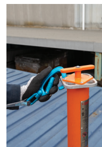
Attach hook on SRL to anchor point on container post
