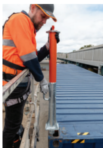
Place container post into ISO corner casting
